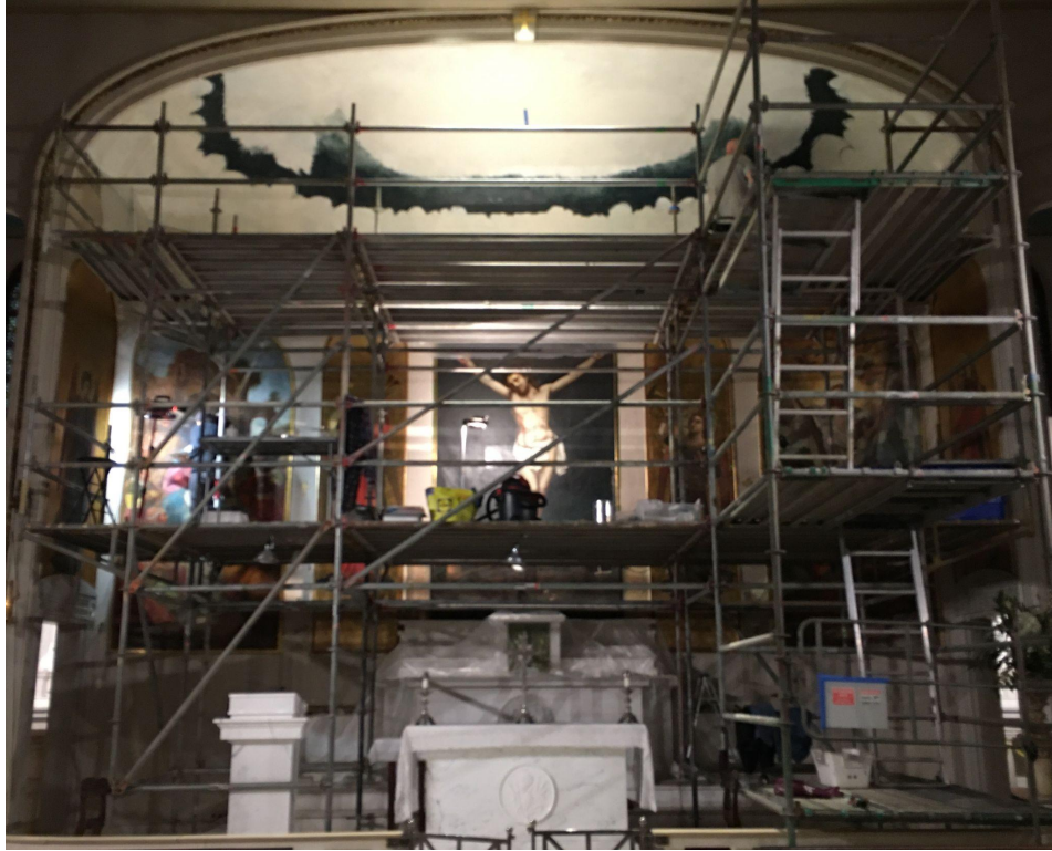
Ceiling Painting in Progress
