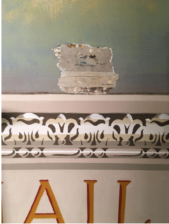
Details of Overpaint Removal & Architectural Design Exposed
