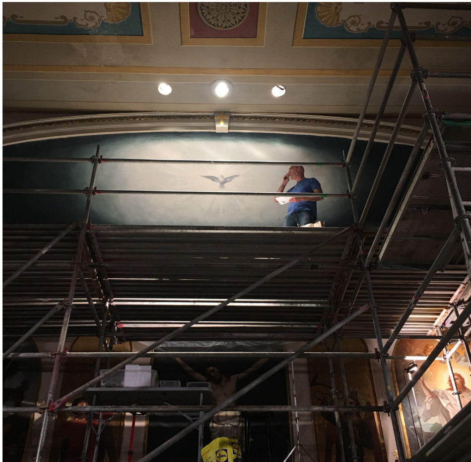
Craig Crawford working on initial Dove design.
