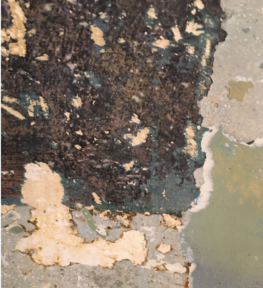
Detail of Overpaint Removal with Light, Medium and Dark Blue Colors Exposed
