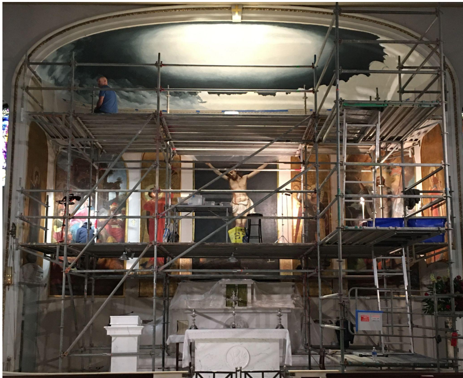
Ceiling Painting in Progress
