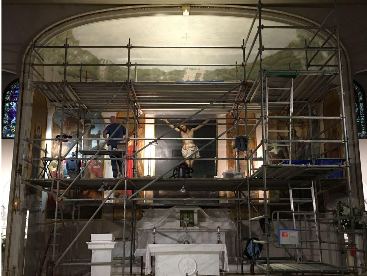
Ceiling Painting in Progress
